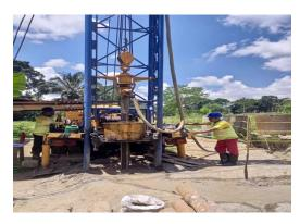
REMADEL's Production Well is expected to yield at least 15 LPS production but during the 72 hours constant discharge test it produces 30 LPS which is more than the expected discharge rate. It will serve approximately three hundred (300) service connections in Brgy. Muaan, Kidapawan City.
